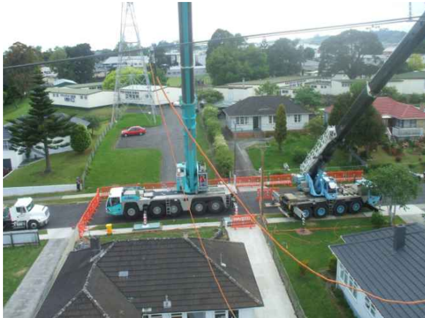
Figure 16: Reconductoring in an urban setting
