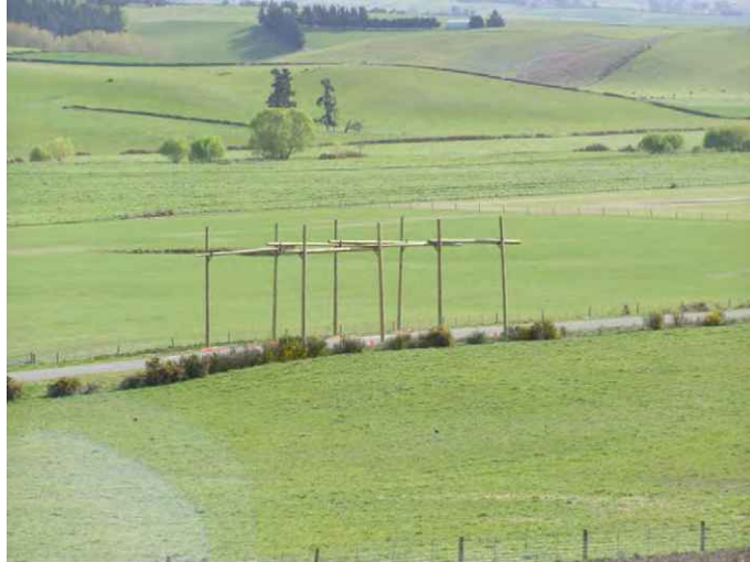
Figure 14: Typical hurdles installed to mitigate potential conductor drop during wiring
