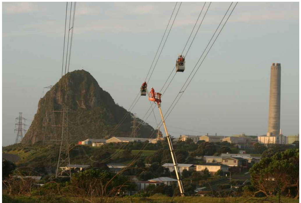
Figure 8: Parallel Body Extension being installed on the BPE-WRK-A line
