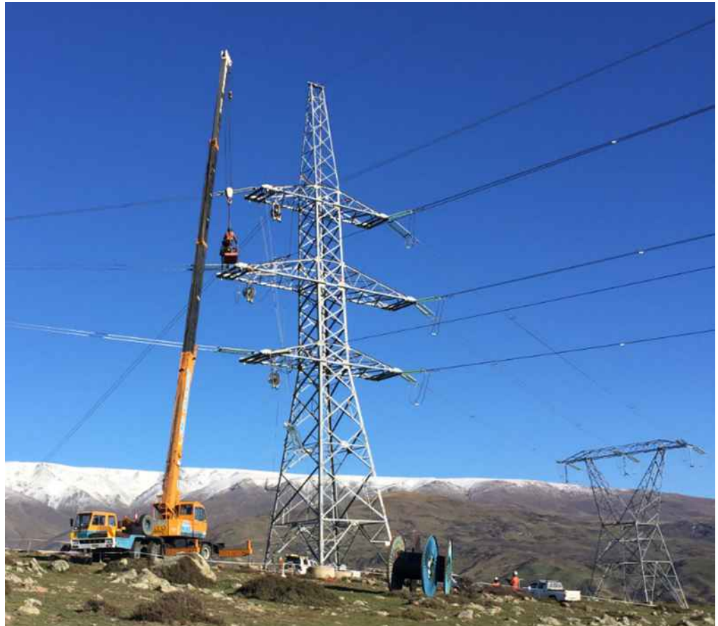
Figure 13: Crane being used for conductor stringing
