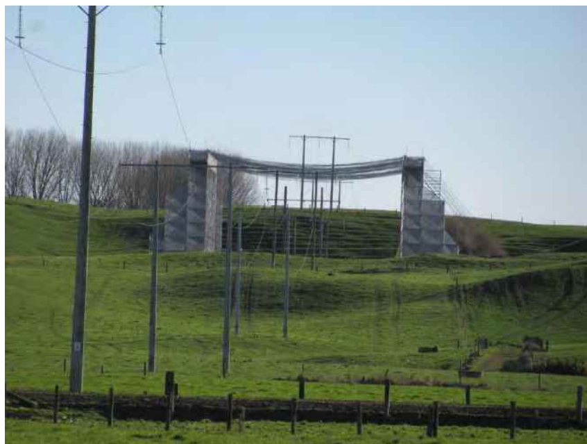
Figure 10: Scaffolding protection structure for stringing
