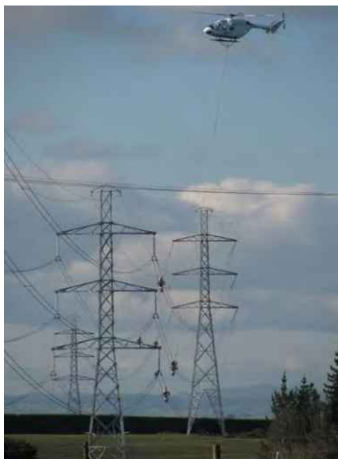
Figure 7: Maintenance work being carried out using helicopters
