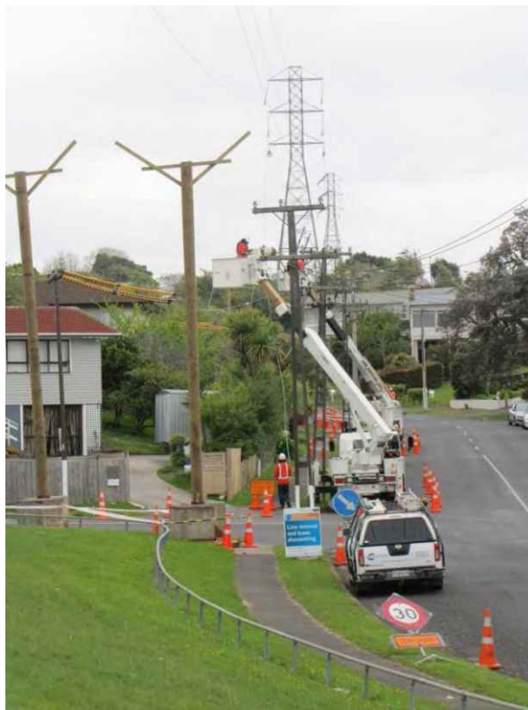
Figure 12: Removal of copper conductor
