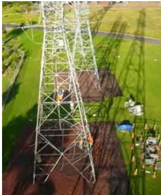
Figure 6: Abrasive blasting in area with no under-build
