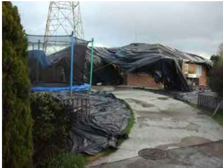
Figure 4: Tower painting in an urban setting, note the extensive polythene sheet protection
