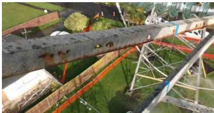
Figure 3: Tower corrosion
