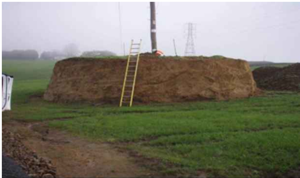
Figure 22: NZECP34 compliant earthworks around a pole on the ARI-HAM-A line
