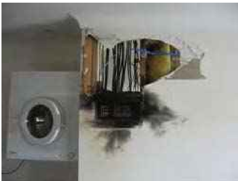
Figure 20: Electrical damage following a conductor drop
