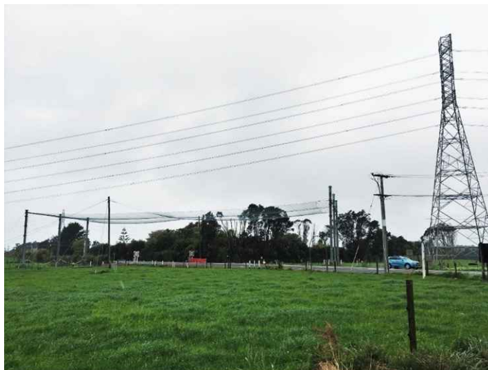
Figure 15: More substantial hurdles installed to mitigate potential conductor drop during wiring
