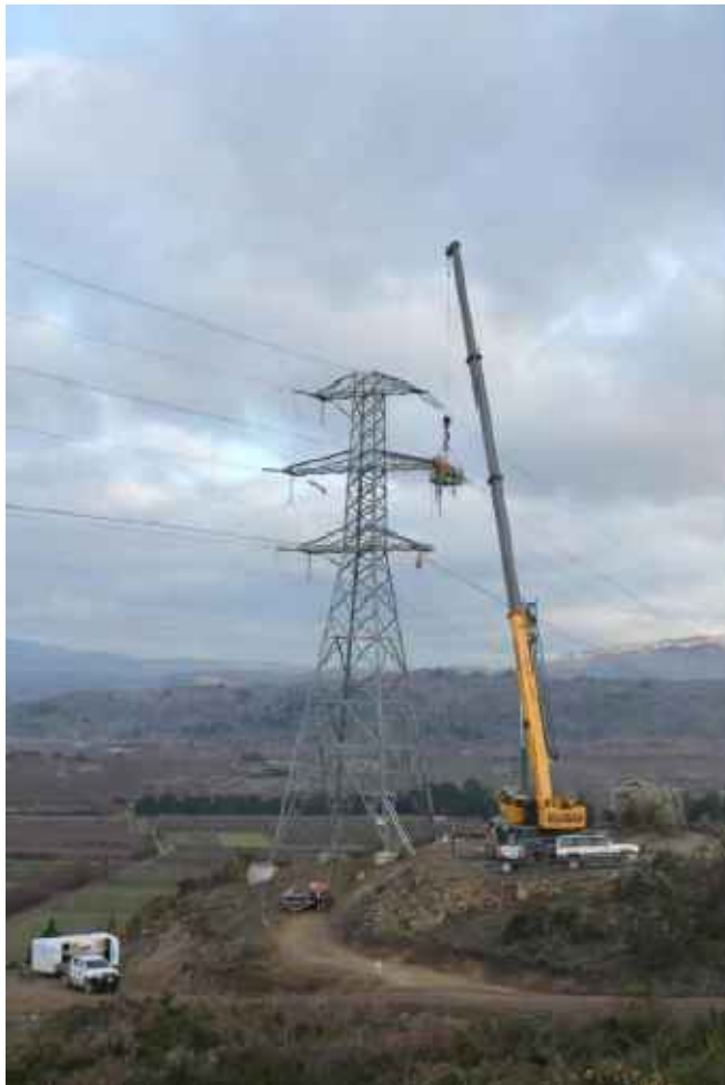
Figure 17: Example crane access required for cross arm and insulator works
