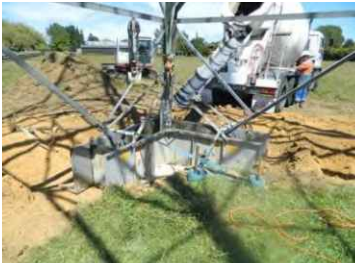
Figure 1: Tower Grillage foundation replacement
