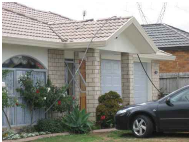
Figure 19: A conductor drop
