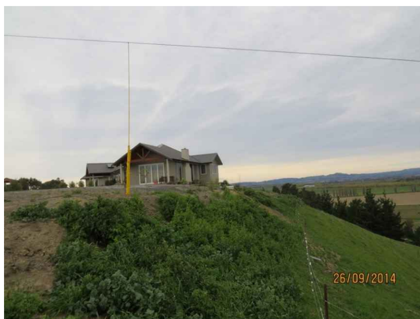
Figure 3: Hastings ground clearance violations
